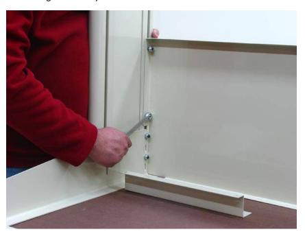
7. Using an electric drill fasten the top of the modesty panel to the bottom of the work surface.
