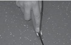
Next, using a Mozart (without the spacer claw), finish trimming the remainder of the weld (image 2). The finished weld should be smooth and on the same plane as the floor covering.
