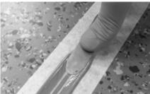
Press the cold weld into the seam using a smoothing spatula, held nearly flat ( $\sim$ 22° angle), resulting in a surface flush and on the same plane as the surface of the tape (image 2). Excess cold weld must be pressed away on each side of the seam. It is important to develop a slight gap between the excess weld and the weld within the seam for easy removal.
